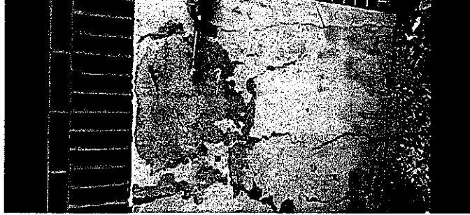
(Delaminated Concrete)
