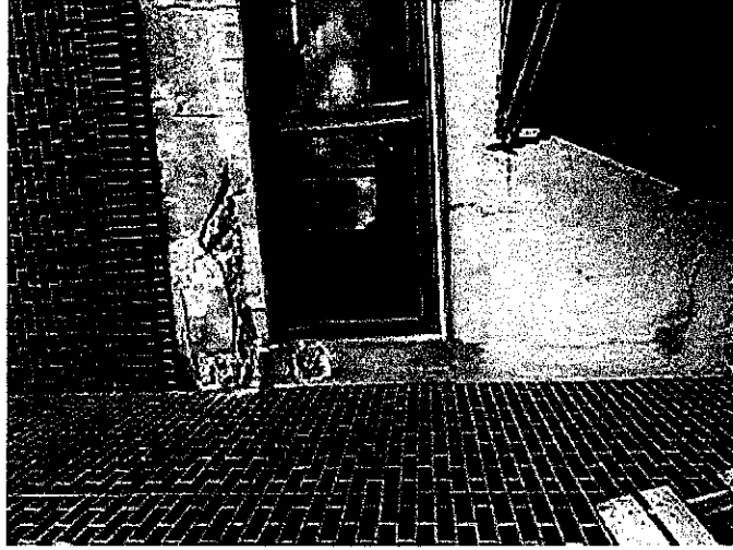
(Additional Spall Repair)
